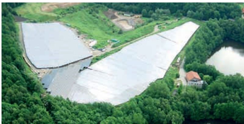
At this PV installation on a former waste tip in Germany the modules form the water-transporting layer. The system was developed by Wagner & Co Solar Technology.
