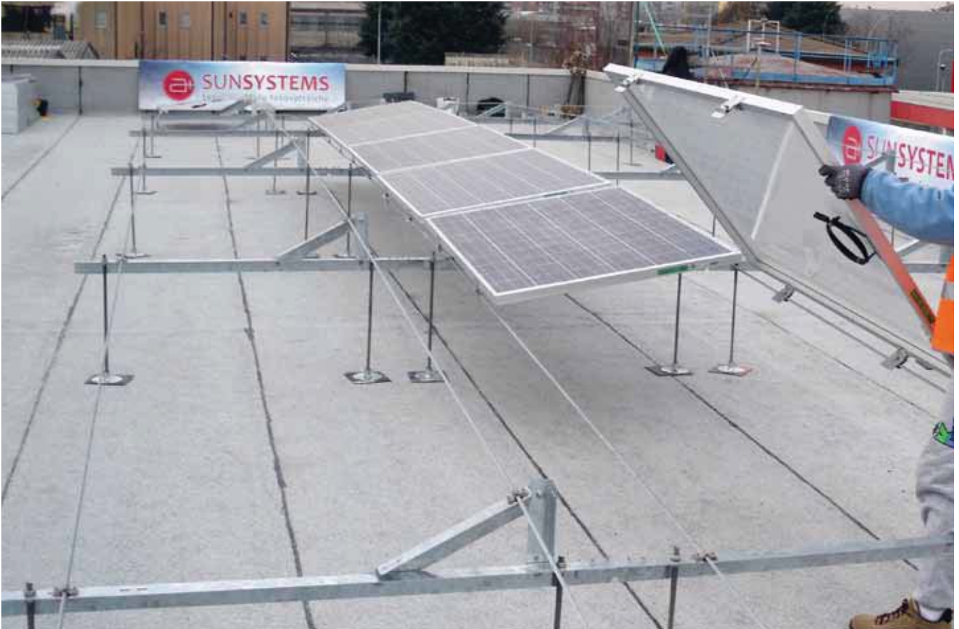
A+ Sun systems' wire rope framing cuts weight in half.
